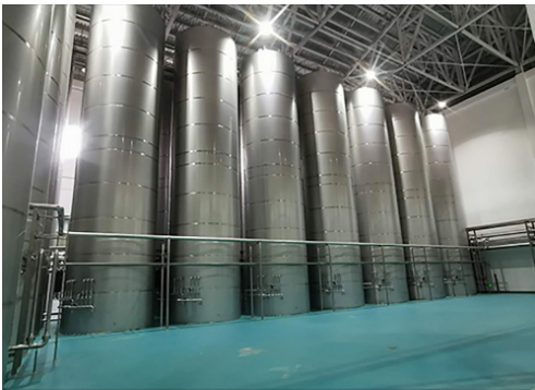
Fermentation Tanks for Condiments
